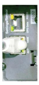
The LAN connection of the UPS Communication interface is connected to the HP LAN switch.
