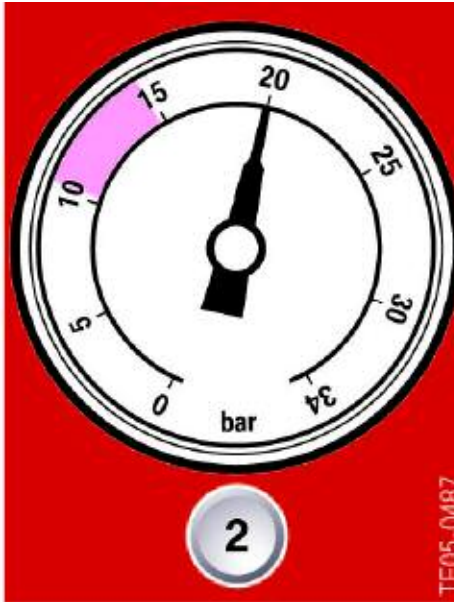
2 = High pressure - too high
